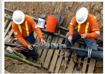
HV Cable Jointers
